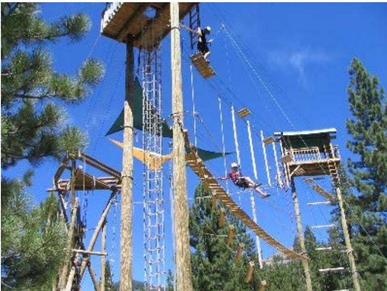
**Figure 3:** A rope course currently in use. Note the way in which the ropes support various structures such as steps and beams and how they connect to the poles. (Ropes course, 2012)
