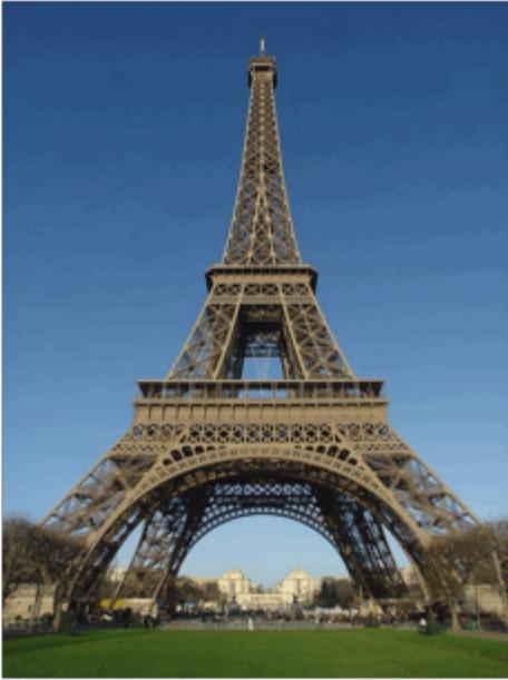
Figure 4 depicts the many trusses composing the framework of the Eiffel tower and how the repeating nature of these simple structures can create the complex tower (EiffelTowerParis 2009).
