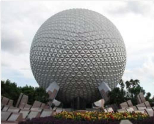
Figure 1-3: The Spaceship Earth is a structure at Disney World’s Epcot Park. This structure is a geodesic dome that is made up of 11,324 individual triangles and follows principle #2 of the “rules-to-build-by” (Morris, 2010). <http://www.csc2.ncsu.edu/conferences/esem/?p=location>
