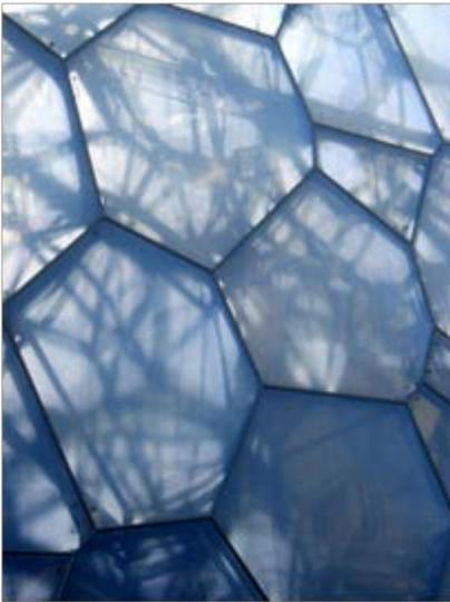
Figure 4: This is a closer look at the cells that make up the water cube. In this image you can see the steel pipes that make the structure, as well as, that ETFE that is stretched over them.
