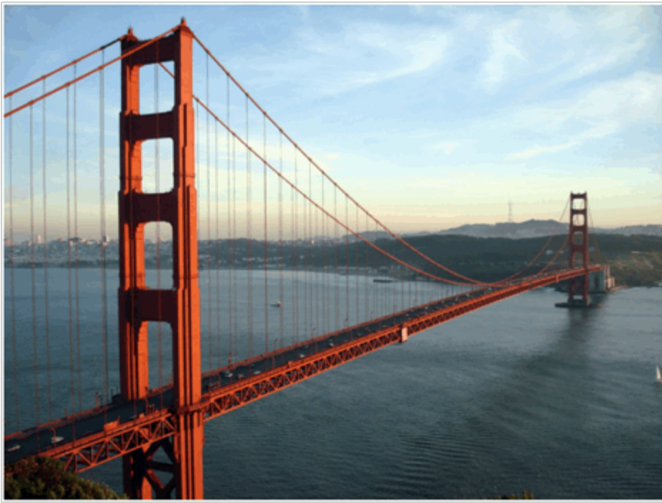
Figure 2: The picture above shows the Golden Gate Bridge, as suspension bridge found in San Francisco, CA. The same structures are seen here as in Figure 1 with the towers, load deck, cables, and anchors (Niewiroski, 2007).
