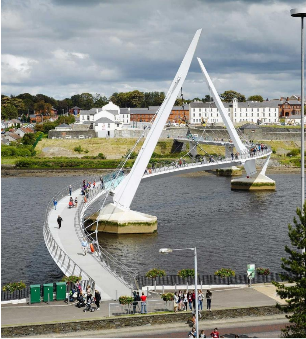
Figure 5: Uniting Forces. Aerial image of the Peace Bridge which looks as though it is one continuous piece, although it is constructed of two identical halves that unite in the middle to form the functional bridge and symbolize unity between the politically divided halves of Derry. (Retrieved from WilkinsonEyre, https://www.wilkinsoneyre.com/projects/the-peace-bridge ).
